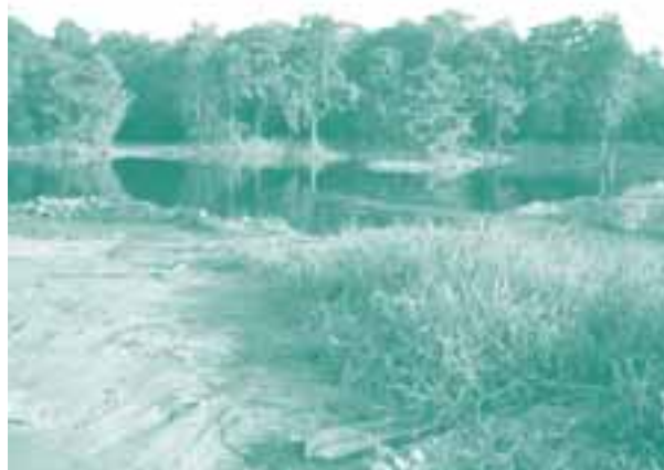
Fish breeding lagoon under construction.
